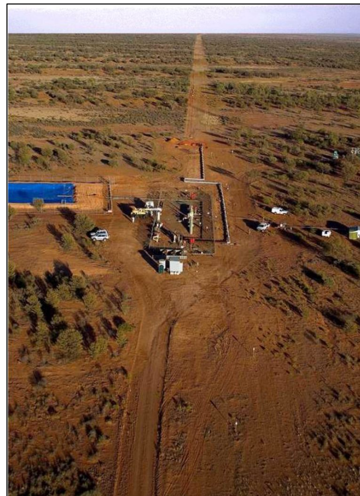
APA's infrastructure is underground and require minimal level of stay-in-business capex
